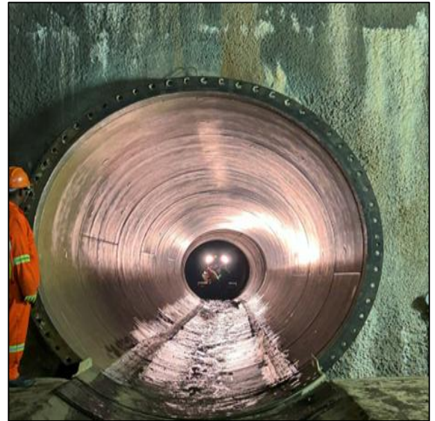
Figure 16: Removing mud inside the tunnel
