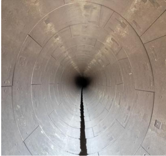
Figure 13: Inside the tunnel
